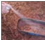
STEP 2: Apply Dust & Dirt Hardener to the surface of the impression.
