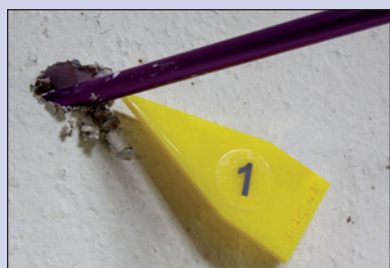
Penetration rod, SirchMark™ marker held by Stikki Dot identifying location and angle of entry
