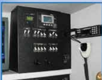
Clearly Labeled Control Panels with Circuit Breaker / Switches to operate and protect on-board equipment.
