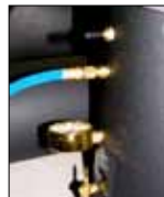
4. Attach one blue hose to the VAC100 Tank.
