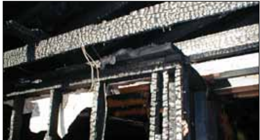
Heavy alligatoring is indicative of intense burning. —Photo courtesy of Franklin County (NC) Crime Scene Unit.
